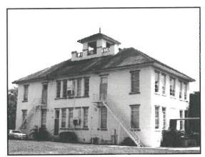
Fig. 47: Original Fire Escape Stairs (National Register Application Form, 1994)
