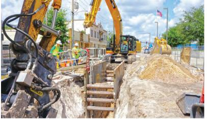
Garney was selected as the design-builder for the upsizing the existing gravity sewer system to provide additional capacity for the City of Orlando's new major league soccer stadium. The project was executed in three phases including:
