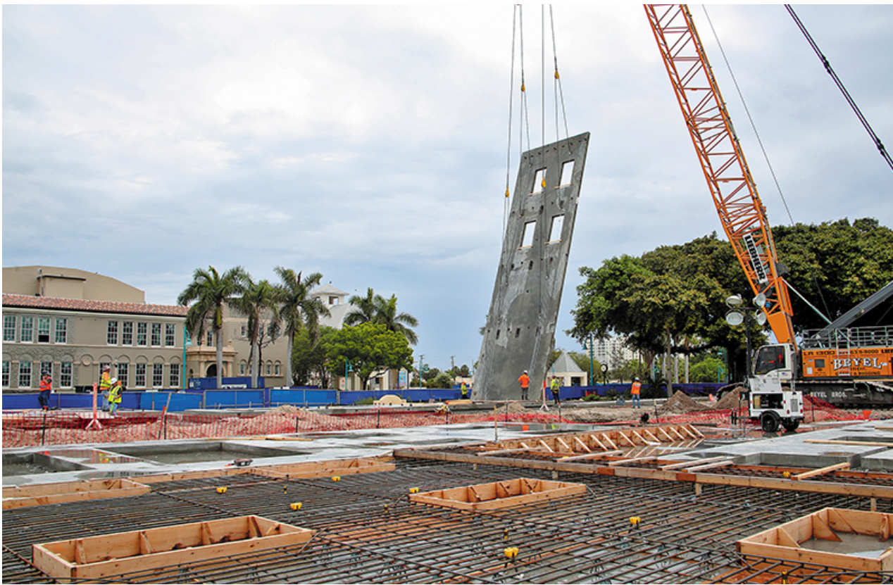
A prefabricated four-story wall is lifted into place at the site of the old community center, across from the restored high school (far left) and Schoolhouse Children's Museum. Tim Stepien/The Coastal Star
